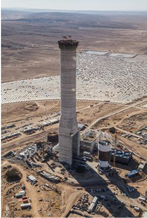
Computers control the system's 50,600 mirrors, which track the sun and concentrate its light on a boiler mounted on the tower. This generates high-temperature steam to power electricity-producing turbines. The plant is being erected by Megalim Solar Power Ltd., a consortium of three companies.
